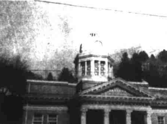
THE "LADY OF JUSTICE" was the victim of strong winds on Tuesday afternoon of last week and came crashing down to the courthouse roof from her perch on top of the dome. The Lady, with her balanced scales, had withstood all kinds of weather for the past 70 years. Her absence leaves a void atop the dome but plans are being made to replace her with a younger lady. (See Heard and Seen column).
