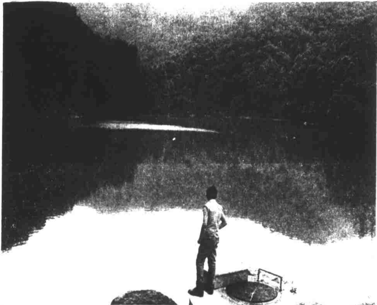
OFFICIALS OF THE TOWN OF MARSHALL have started lowering the water level in the reservoir which supplies the town with water in compliance with an order by the N.C. Environmental Management Commission, which contends that the
