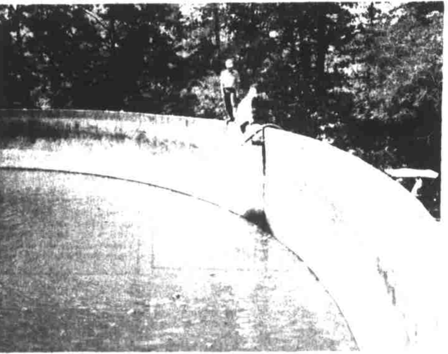
MEMBERS OF THE FRENCH BROAD EMC are also assisting in the operation. Pictured above looking at the water being released into the reservoir are Randy Roberts (standing) and Howell Cody (sitting.) It can be noted that the million-gallon reservoir is dangerously low of water due to having to abandon the storage lake on Hunter Creek, the lowering of the lake by a foot a day, and the extended dry spell, despite needed rains over the weekend.
