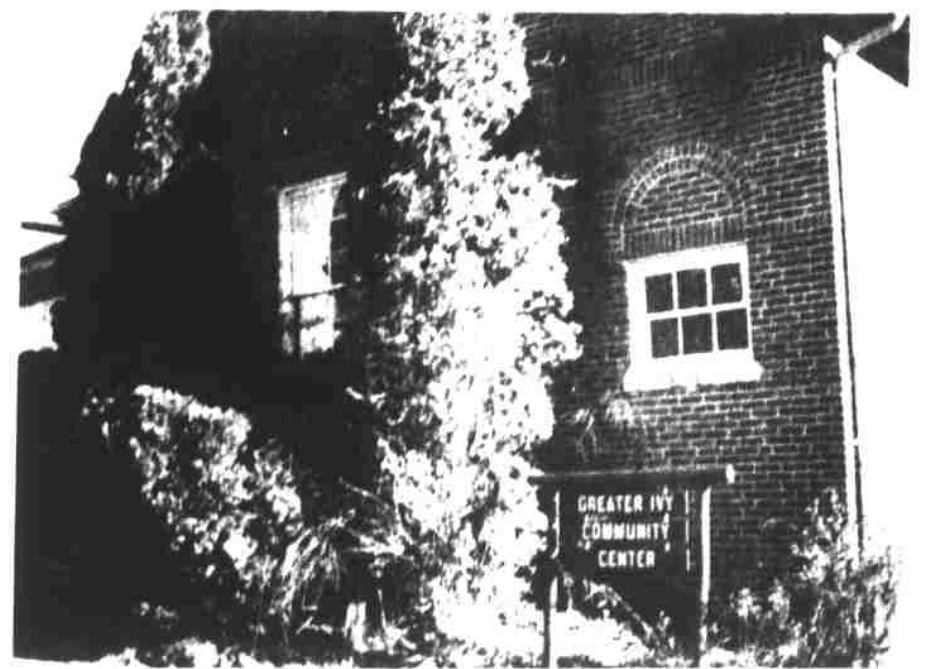
GREATER IVY COMMUNITY AND RECREATION CENTER (FORMER BEECH GLEN SCHOOL)
