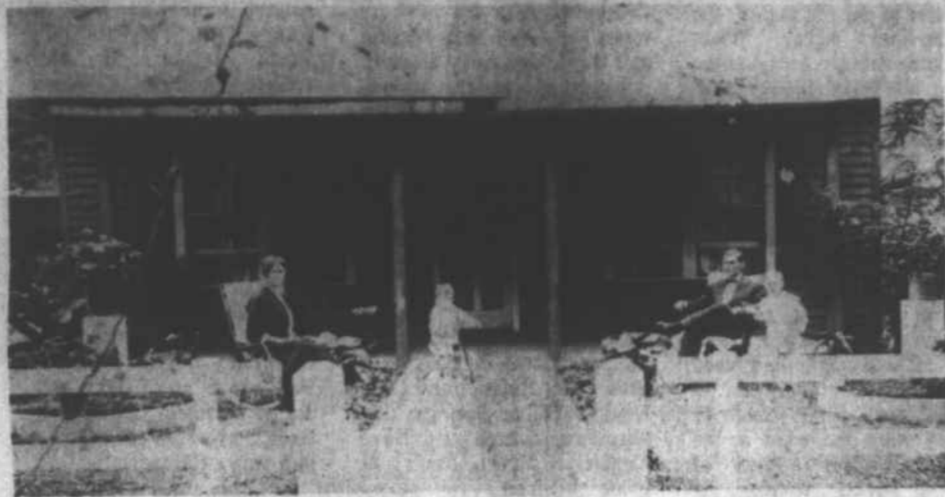
PICTURED ABOVE is the residence of the late Mr. and Mrs. W.I. Tweed which was located on Main Street in Marshall where the Ponder Auto Supply Co., is now located. The picture was made prior to 1916 when the house was washed away in the 1916 flood. Shown, left to right, Mrs. Tweed, Leslie Tweed (on tricycle) Mr. Tweed and son, Connor (deceased). Leslie, of Marshall, is the only surviving member of the immediate family. A freight car on railroad can be seen at extreme left.
