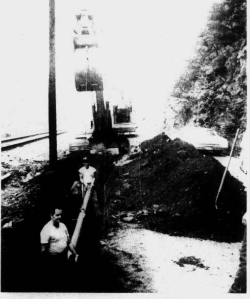
NEW six-inch water lines are being installed beside U.S. 25-70 and the Southern Railway from the Marshall depot to a point opposite the Fortner property where the new pipe will go under the railroad and river to the wells recently dug. In the next several months the pipe will be installed down Main Street and a connector
