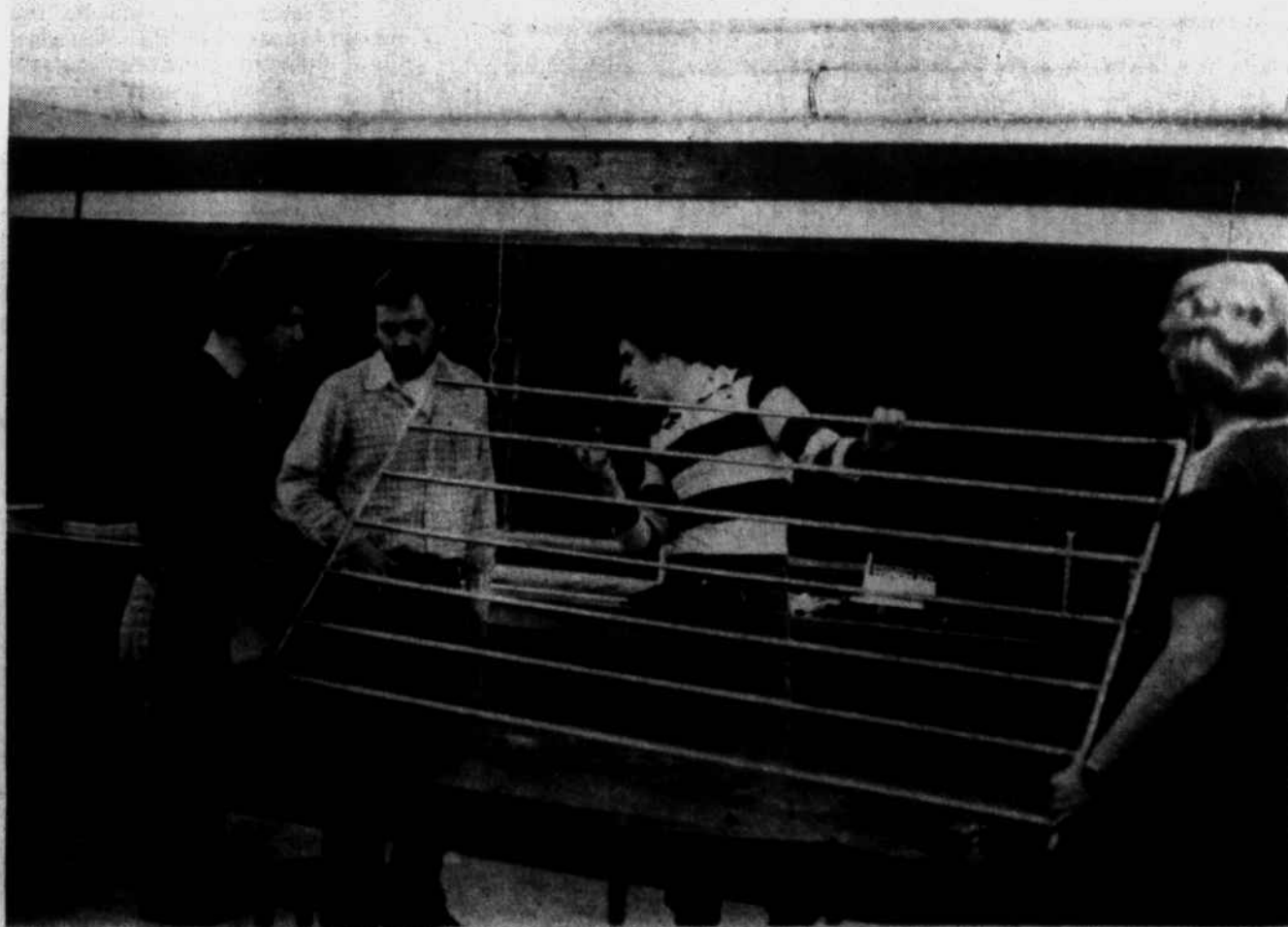
SOLAR ENERGY classes at Mars Hill College proved highly successful as shown above as students construct a manifold hot water collector. Plans are being made to resume the solar heating classes at the
