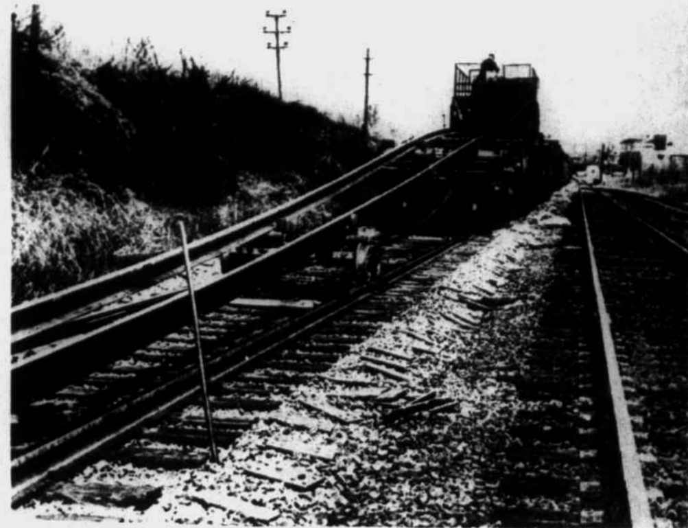
CONTINUOUS welded rails are now being installed by Southern Railway System (shown above), which, among other improvements, will eliminate the familiar "clickety-clack" sound by train wheels crossing crack joints.
