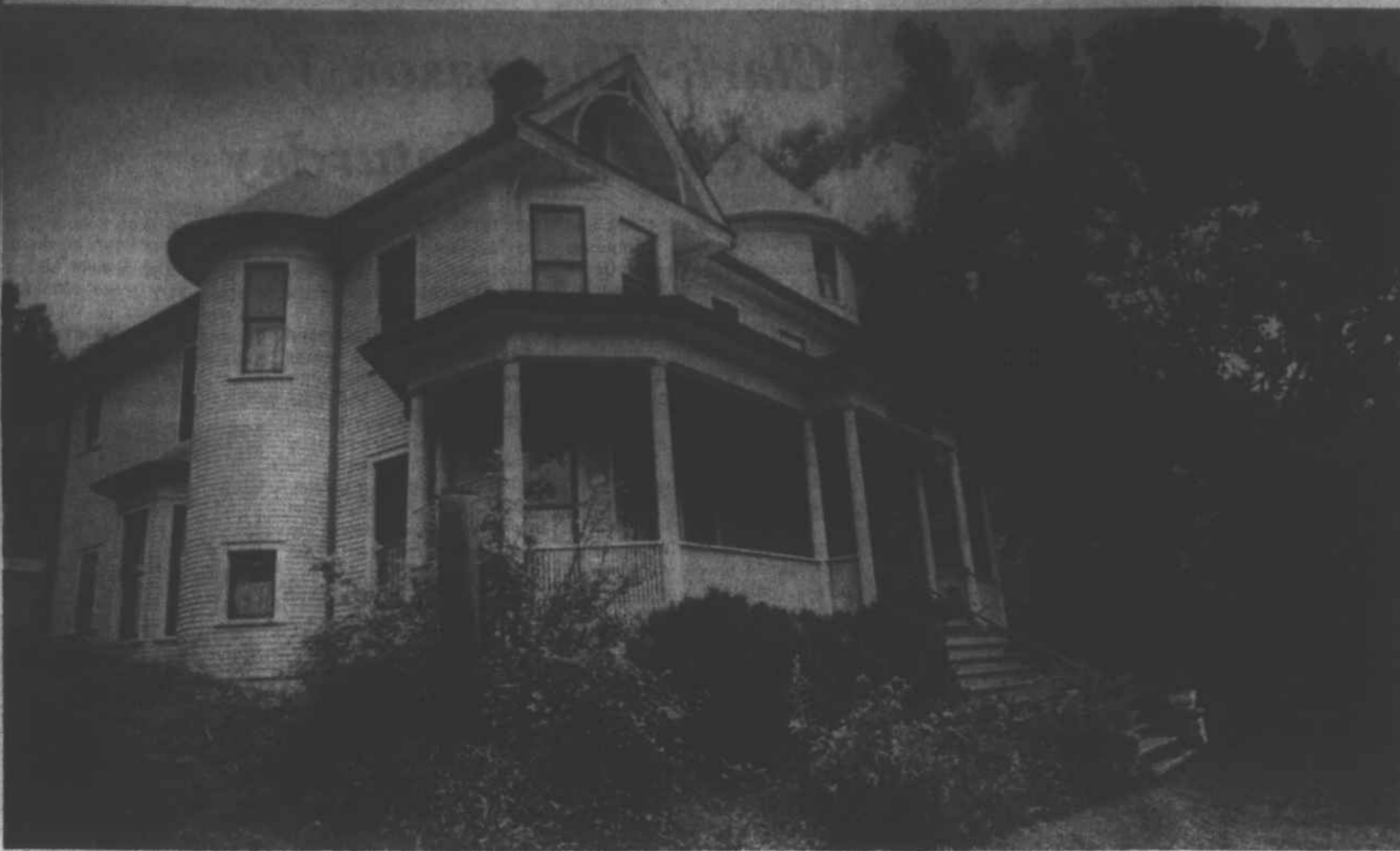
A mountainside was cut out with pick and shovel to build the Stackhouse residence.
