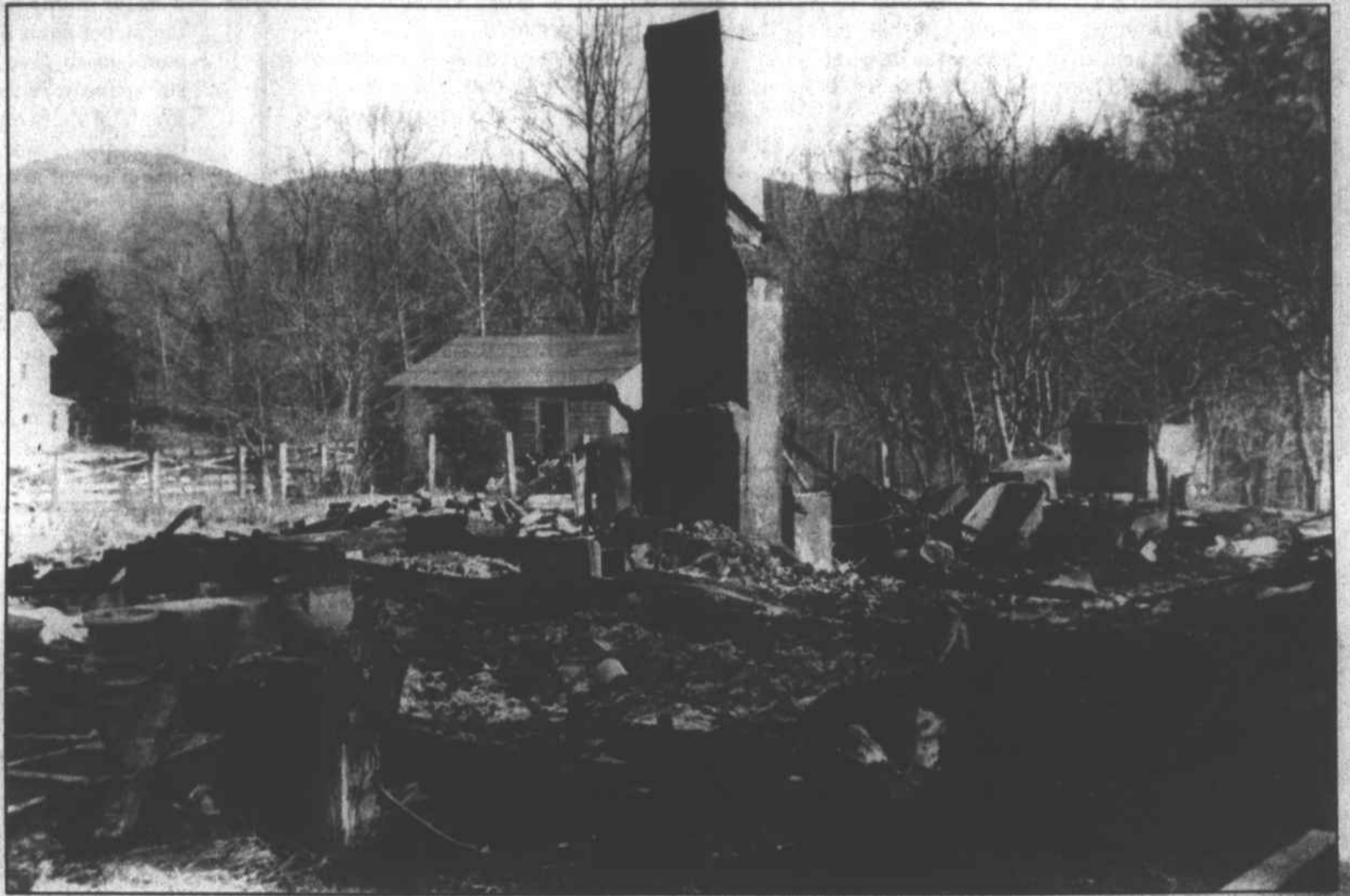
Only Chimneys and Foundation Remain At Home Of Hank Holmes
