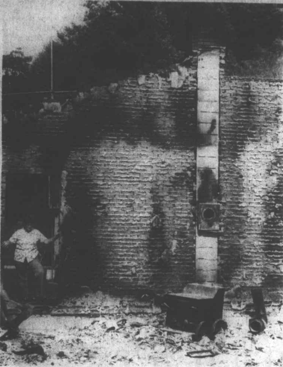
NEIGHBOR Cosie Ray looks over stove and flue believed to have caused the Shelton Laurel fire.
