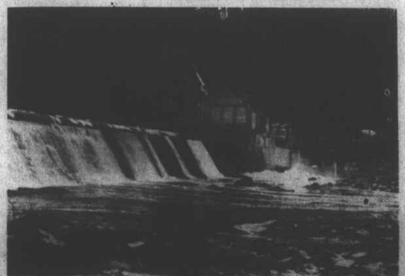
REDMON DAM AS IT APPEARS TODAY, ready to return to service at five times its original capacity.
