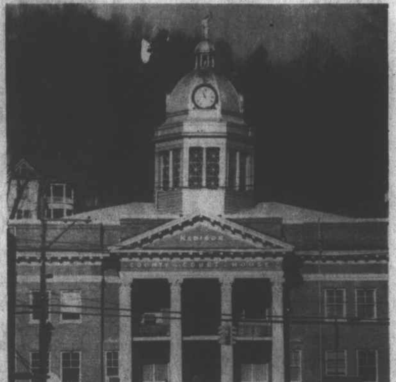
REPAIRS TO THE MADISON COUNTY COURT HOUSE WILL FORCE CANCELLATION of court sessions, possibly as late as April, officials were told last week. Photo by Bob Koenig
