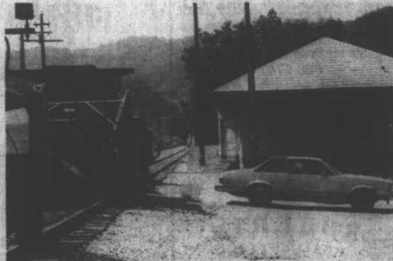
MARSHALL'S RAILROAD DEPOT
