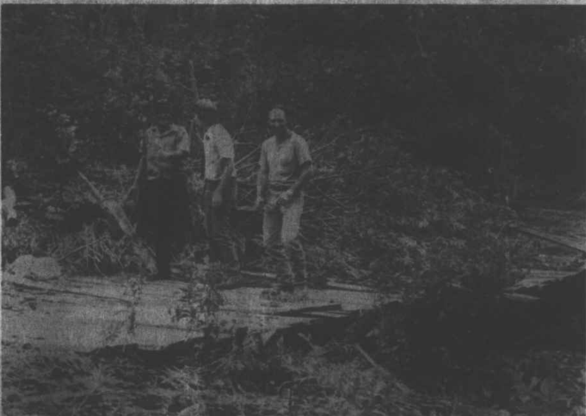
Big Pine Residents Survey Flood Damage To Bridge
