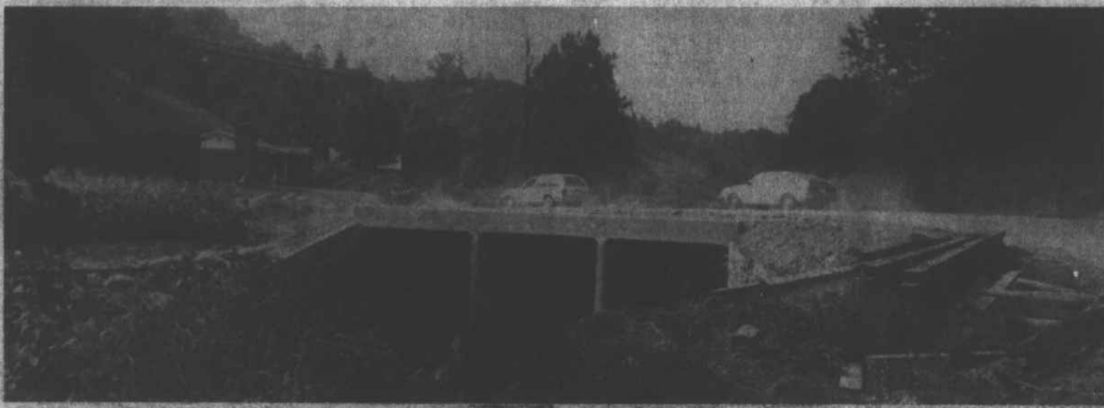
Grapevine Road has a new bridge and is now open for traffic.
