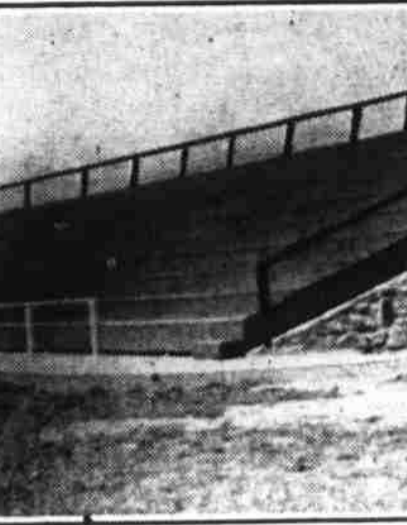
This is the new Township stadium, recently completed at a cost of $8,000. It will seat over 1,500 comfortably and will be dedicated at 8 o'clock Friday afternoon before the Waynesville-Sylvia game. The stadium is a WPA project.
