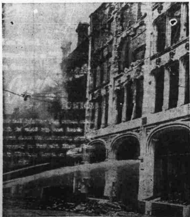
Firemen play their hoses on the smouldering wreckage of a building in London after a German bombing raid which caused widespread damage to the British capital. Photo was flashed by cable to New York.
