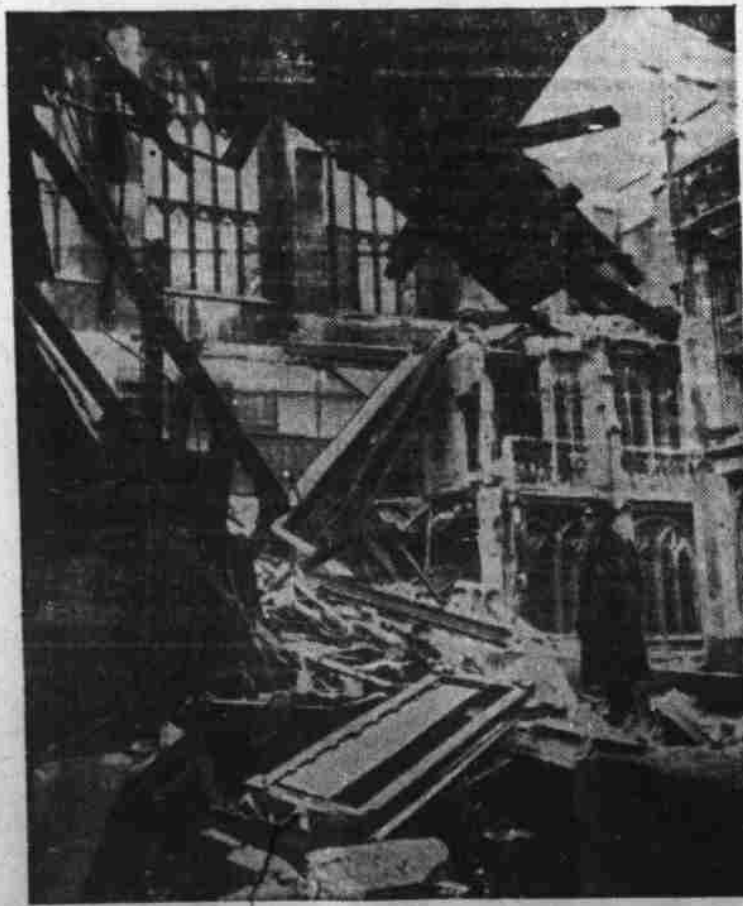
Here is a view of the damage caused when a German fire-and-explosive bomb struck Britain's historic Parliament building in London within a few yards of the House of Commons chamber. The blast wrecked the 600-year-old St. Stephen's Cloisters and did other extensive damage. Parliamentary staff members were in shelters and no casualties were reported. Fires were extinguished within half an hour.
