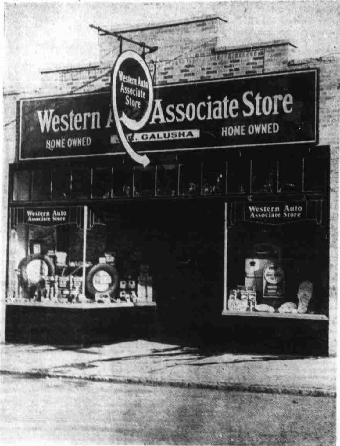
The new building, located on the Willis Property on Main Street, recently built and now occupied by the Western Auto Associate Store, owned by Mr. and Mrs. James C. Galusha.
