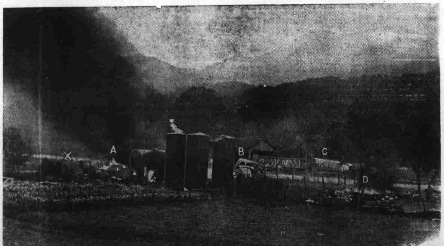
This photograph was made from the back of the C. M. Dicus residence and shows the area damaged by the two explosions at the Standard Oil bulk plant here Tuesday morning. "A" is burning oil that was stored in the warehouse. The white flame can be seen leaping from the upright tank on the left. "B" is the remains of the transport truck, which was loaded with 4,000 gallons of gasoline and exploded thirty minutes after the tank "C" was blown across the street, the car and the double railroad track. The tank (C) was a twin tank to the horizontal tank and was about where the letter "A" is when it exploded. "D" is the ruins of the Caldwell home, where three died. "X" is where the Paul Walker home was blown down and burned. All vegetation for hundreds of feet was as brown yesterday as if it were midwinter.
