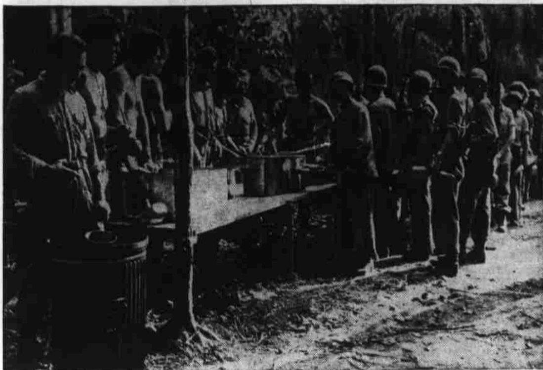
Between forays against the Japs on Guadalcanal in the Solomons, U. S. marines line up at a field kitchen for a hot meal. The navy reported that a Jap feeler thrust against the western flank of American positions guarding the vital airport on the island had been repulsed. U. S. planes are still taking off from the field to bomb enemy troops and supply concentrations. This is an official U. S. Marine Corps photo.
