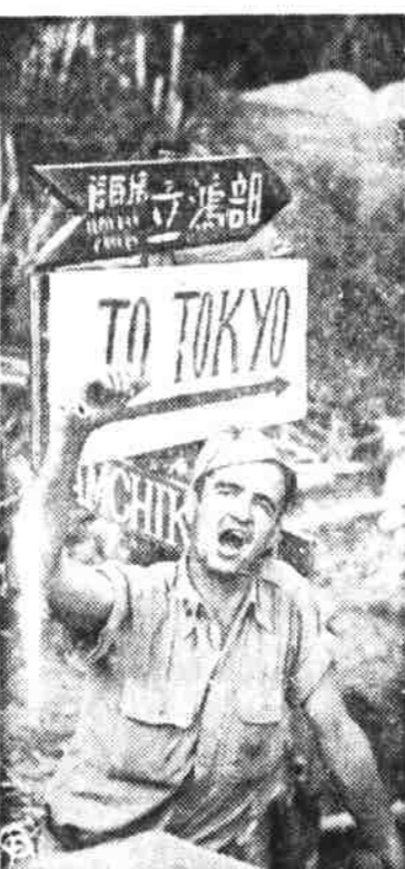
CAPT. JOHN E. MOYER of Tuskegee, Ala., is highly confident in this picture that the road he is helping to build near the Burma border will eventually lead to Tokyo. He is one of the Army engineers working on the project. (International)
