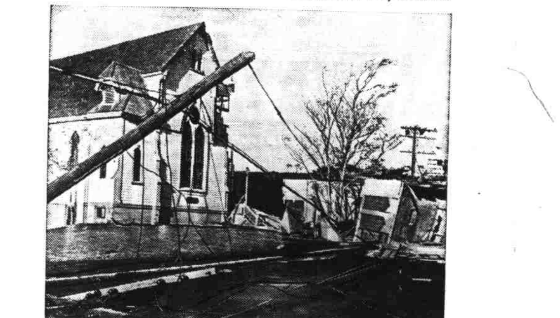
The big blow twisted the steeple off this Massachusetts church and toppled it into the street across the electric wires. Another headache for hard-working linemen!
