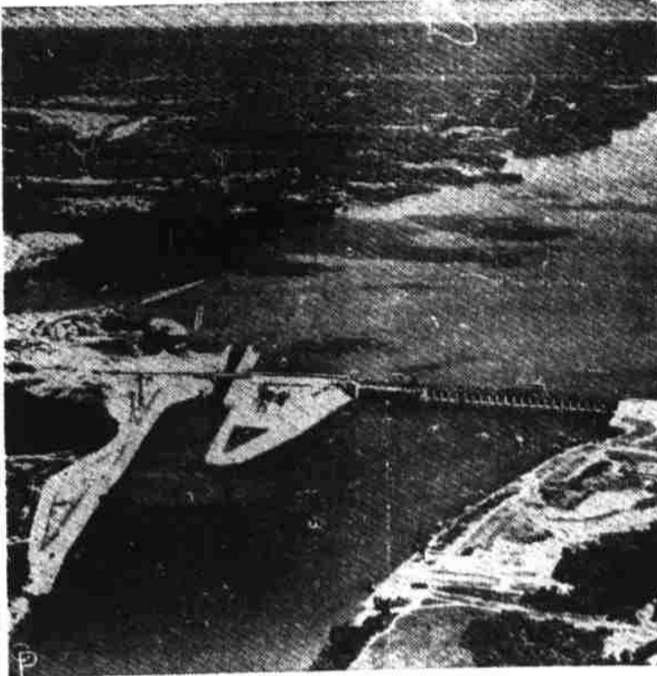
THIS NEWEST TVA DAM, on the Tennessee River near Paducah, Ky., to be dedicated Thursday by President Truman, serves the multiple purpose of aiding navigation, controlling floods and supplying power. The dam will impound four million acre-feet of flood storage; will create a deep river navigation channel 184 miles long and will generate one hundred thousand kilowatts of electrical power. (International)
