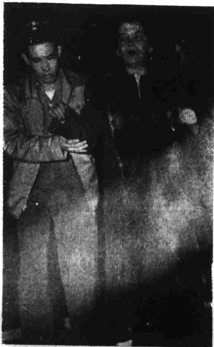
An unidentified and frightened woman guest at the Winecoff Hotel is led from the smoke and flame-filled shell of the building by a taxicab driver early Saturday morning. More than a hundred were killed—Atlanta Constitution photograph.
