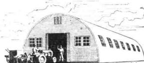
QUONSET 40-40 feet wide by any length desired in sections of 20 feet. The standard building has big-double, free-sliding steel doors, four steel windows and large, adjustable ventilating louvers in each windows for side walls and solid end walls are also
