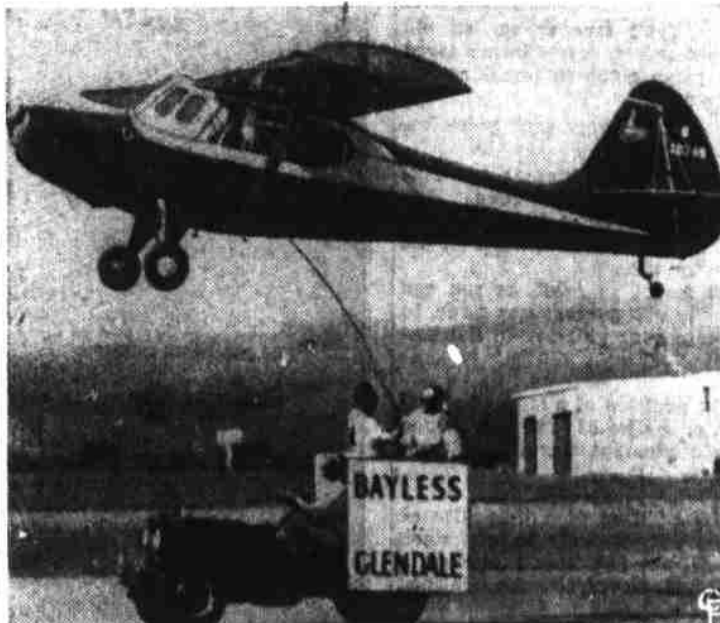
GOING THROUGH their refueling procedures, fliers Bill Barris and Dick Reidel make practice runs for their scheduled attempt to break the light airplane endurance flight record. The gasoline, in five gallon cans, is hauled into the plane from a jeep traveling up and down the airstrip. Other supplies will be conveyed in similar fashion. (International)
