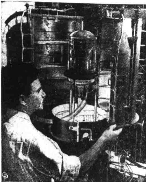
STANDING ON A PEDESTAL in Pittsburgh is the first working model of an X-ray "telescope," or image amplifier as it is technically known...
