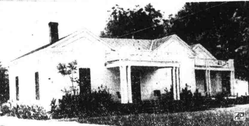
The ramshackle house (top) was just another old eye-sore until a remodeling job converted it into the attractive home (bottom) of Mrs. Dorothy Webb, winner of a community home improvement contest at Macclesfield. The town, once dingy and dirty, with unpainted buildings and abandoned, rotting shacks, has won $2,000 in cash prizes offered in a magazine contest for the nation's best job of community beautification. (AP Photo)
