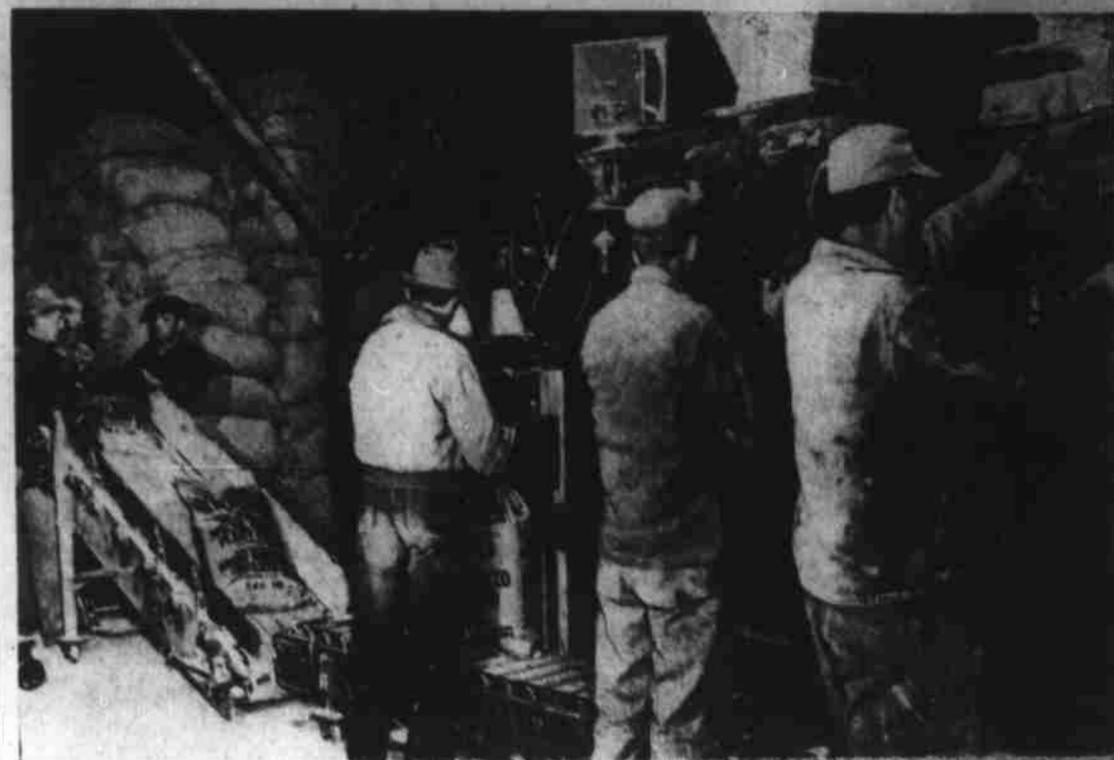
Two automatic machines fill the specially made paper bags with an even 100 pounds net of Plant Food. The two men at the right are filling bags, while the third man is operating the sewing machine which sews the tops of the bags. Then the bags go to the conveyor, left, and on to storage, or direct into waiting trucks. Automatic scales are attached to each filling machine to assure accuracy. (Photo by Ingram's Studio.)
