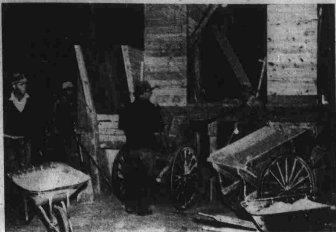
Workmen are shown here pushing carts and wheelbarrows of different materials used in making Plant Food. All materials are dumped into a pit, and from there it is carried by chain buckets to the third floor for mixing and grinding. All materials are carefully weighed and analyzed before going into the mixing machinery. (Photo by Ingram's Studio.)
