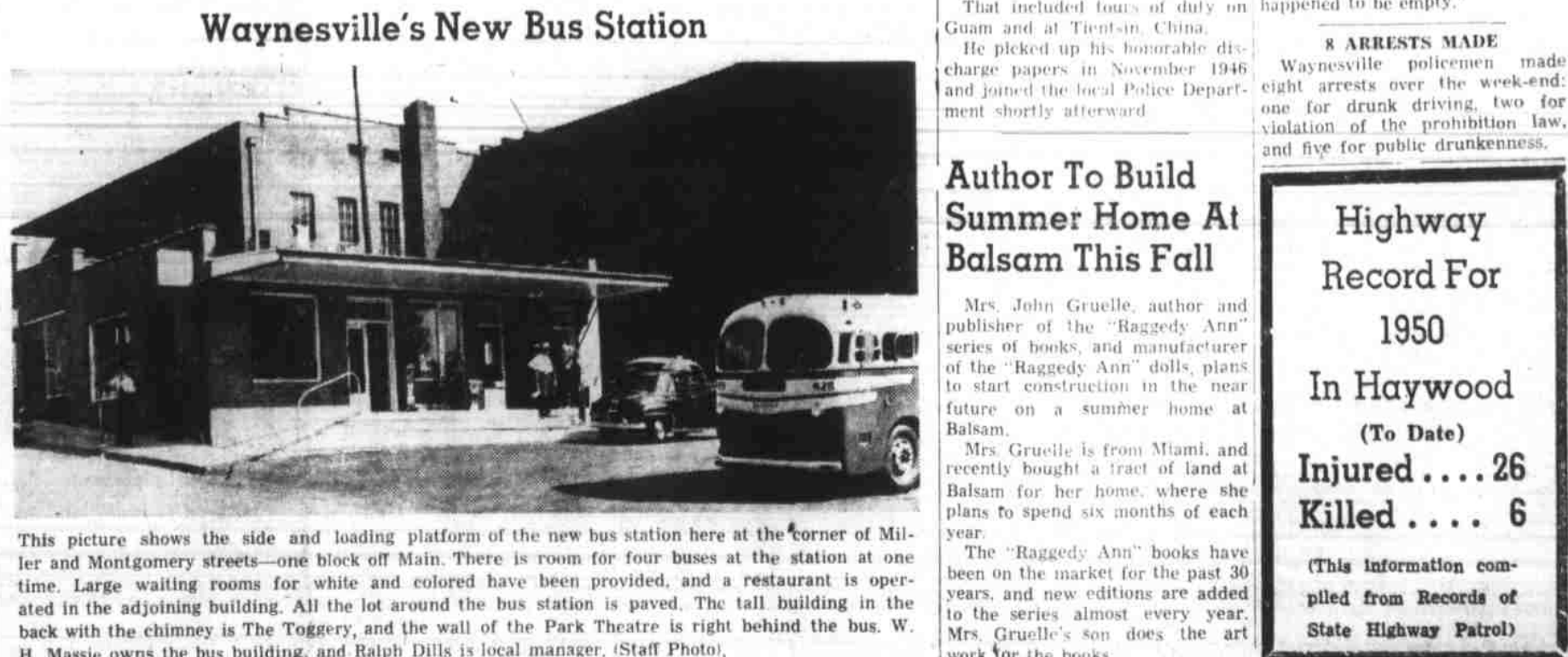
This picture shows the site and loading platform of the new bus station here at the corner of Miller and Montgomery streets—one block off Main. There is room for four buses at the station at one time. Large waiting rooms for white and colored have been provided, and a restaurant is operated in the adjoining building. All the lot around the bus station is paved. The tall building in the back with the chimney is The Toggery, and the wall of the Park Theatre is right behind the bus. W. H. Massie owns the bus building, and Ralph Dills is local manager. (Staff Photo.)
