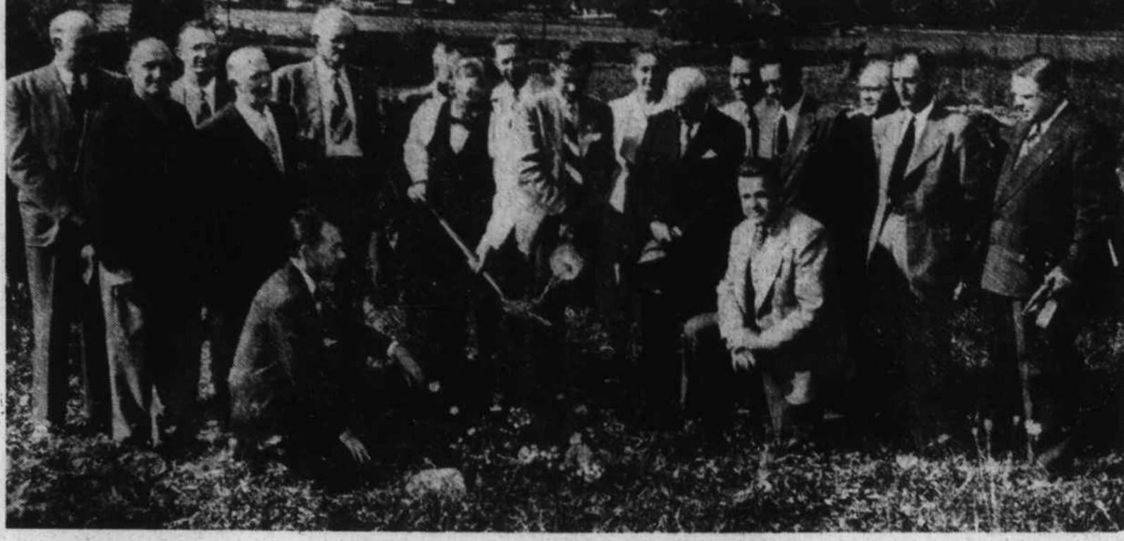
J. W. Killian, chairman of the board of education, turned the first shovel of dirt, to formally break ground for the modern vocational building at Waynesville high here Wednesday afternoon. Officials and civic leaders looked on as the ground was broken. Kneeling, left, M. H. Bowles, district superintendent; right, C. E. Weatherby, high school principal. Standing, left to right: W. Roy Francis, county attorney; Guy Massie, member school board; James Noland, member of the board; Jarvis H. Allison, commissioner; Charles C. Francis, chairman board of commissioners; Mr. Killian; Jonathan Woody, president, First National Bank; Harry Robinson, Jaycees; Dave Felmet, chairman of advisory committee, and representing Rotary; Mrs. Lucy Jones, county superintendent of education; Mayor J. H. Way, Waynesville; Jimmy Childress, Kiwanis; L. C. Davis, mayor of Hazelwood; John B. Smith, Boosters Club; Lee Davis, Lions Club, and W. Curtis Russ, editor The Mountaineer. (Mountaineer Photo).
