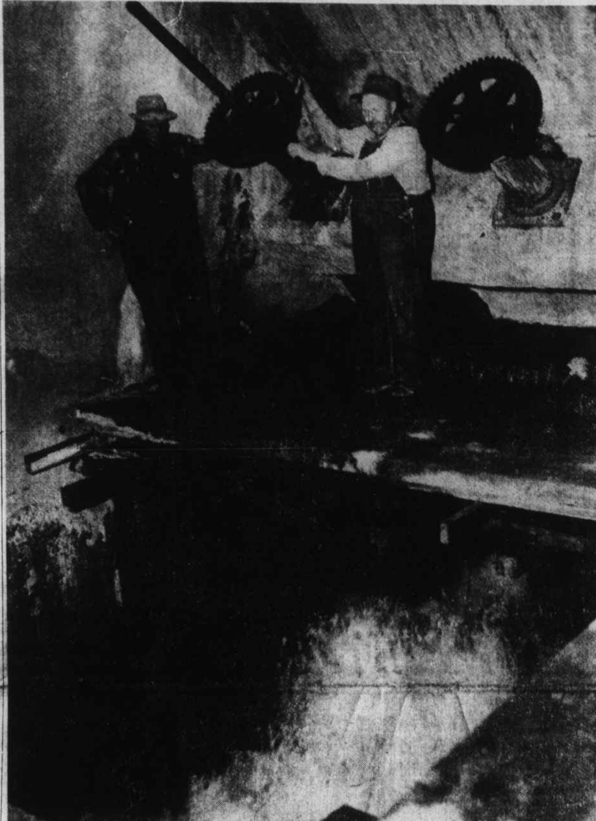
The water level of Lake Junaluska was lowered over the week-end by the opening of the flood gates. The water will be kept down about 7 feet for several months for a major dredging job of the upper part of the Lake, and the construction of a modern sandy beach. On the left, M. H. Gaddis, grounds foreman, and his assistant, Frank Smith, are shown opening the flood gates to lower the water level. (Mountaineer Photo.)
