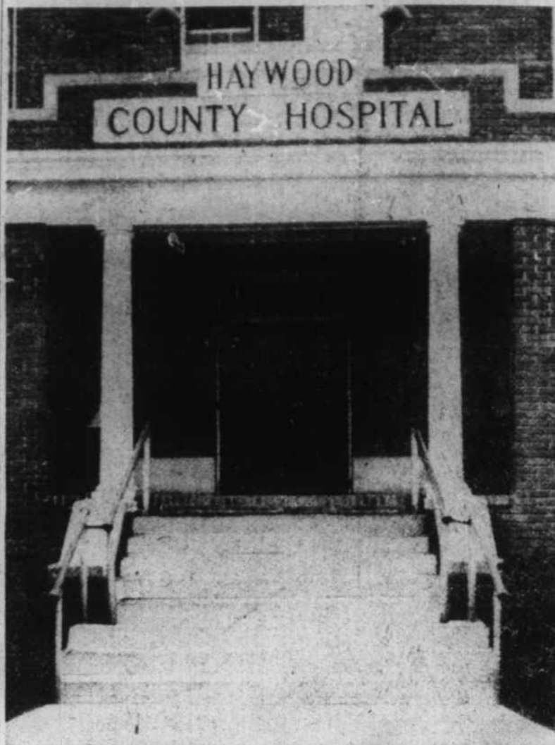
This is the familiar entrance, which has been used for the entire 25 years the institution has been built. No changes were made during the modernization program to the entrance, except for a repainting job. (Mountaineer Photo).
