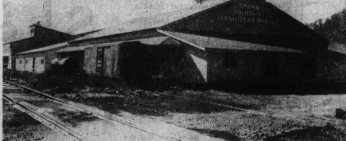
THE SECTION'S NEWEST industrial plant is the Western Carolina Phosphate Company, adjoining the Smoky Mountain Fertilizer Company, just south of Hazelwood. The new plant is beyond the tank car on the side track. The owners of the Phosphate plant also own the Fertilizer plant. Production will get under way on Monday. (Mountaineer Photo).
