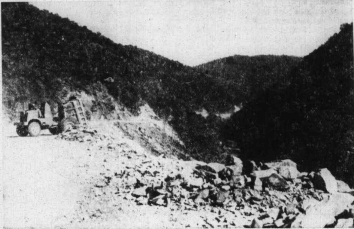
THOUSANDS OF TONS OF ROCK complicate the task of carving the new Pigeon River Road from the mountainside in the Waterville section of Haywood County. Here a truck dumps a load of rocks and dirt from a steam shovel at work on the road. (Mountaineer Photo).
