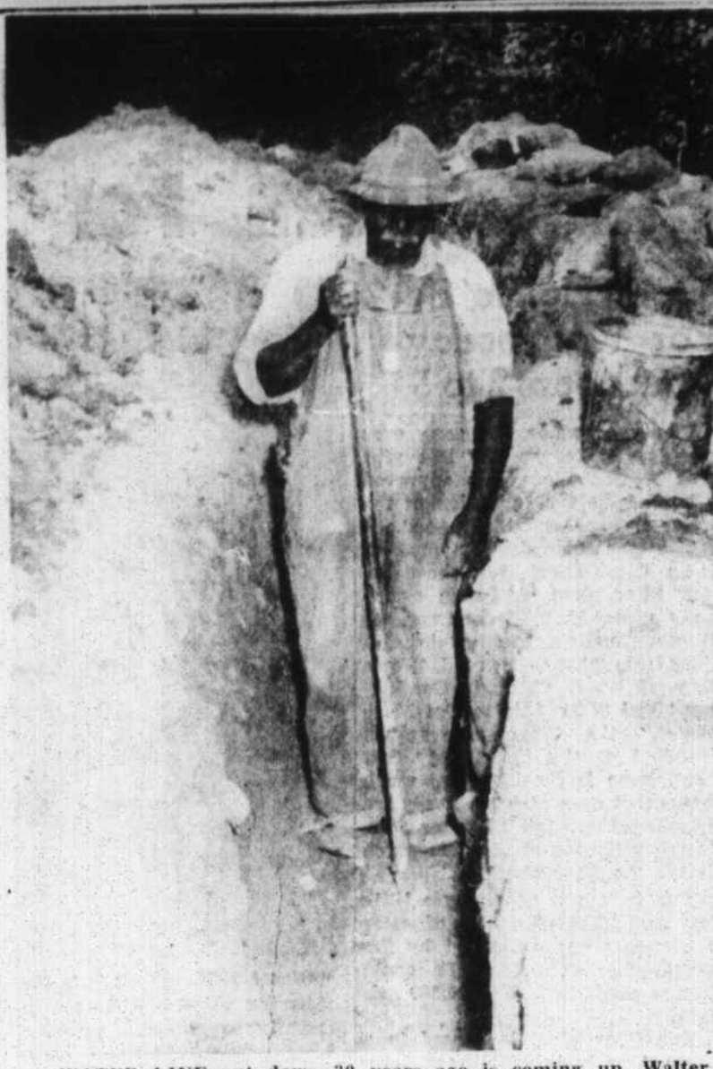
A WATER LINE put down 30 years ago is coming up. Walter Haley, member of the town water repair crew, is shown on the Waynesville Water Shed, taking up a mile of cast iron pipe which is as good as new pipe. Bradford Mehaffey, superintendent said. The pipe will be used in a new line, saving the Town thousands of dollars, the officials said. (Mountaineer Photo).
