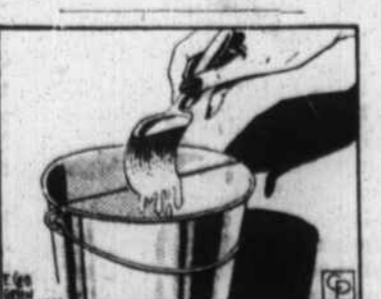
For indoor painting chores, mix the paint in a galvanized steel pail to prevent splattering. Next stretch a wire, fastened to the pail's handle attachments, across the top of the pail and use it to remove excess paint from the brush during painting.
