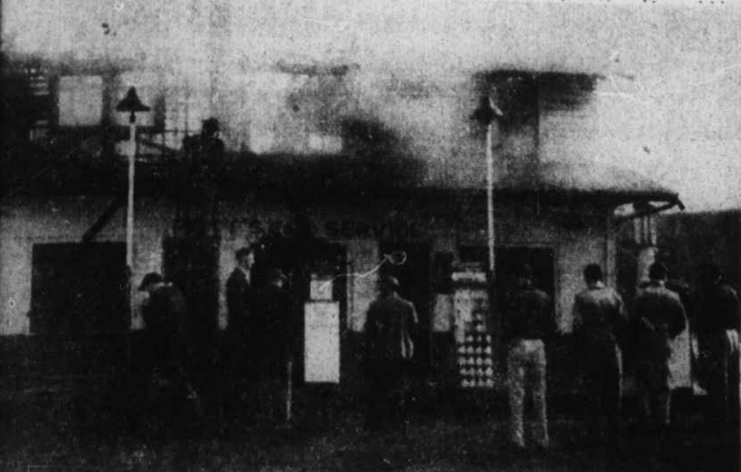
ESTIMATED AT $11,000 was caused by a fire which swept through the story of the Ed Potts service station at Lake Junaluska—ignited by a defective flue
