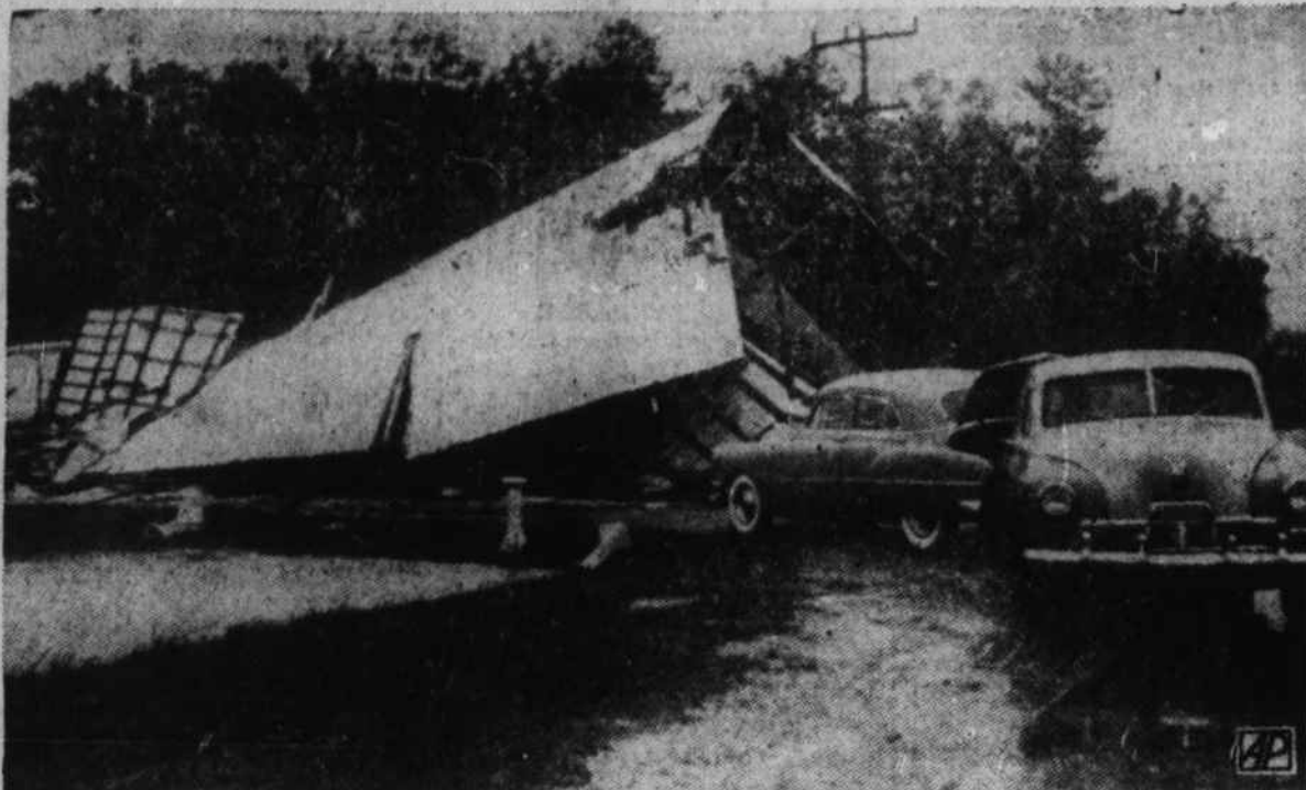
HURRICANE IONE leaves trail of wreckage. Salvage workers pull an automobile from the wreckage of a drive-in theater near New Bern, after hurricane Ione slammed into the coastal area, doing damage that runs into millions of dollars.
