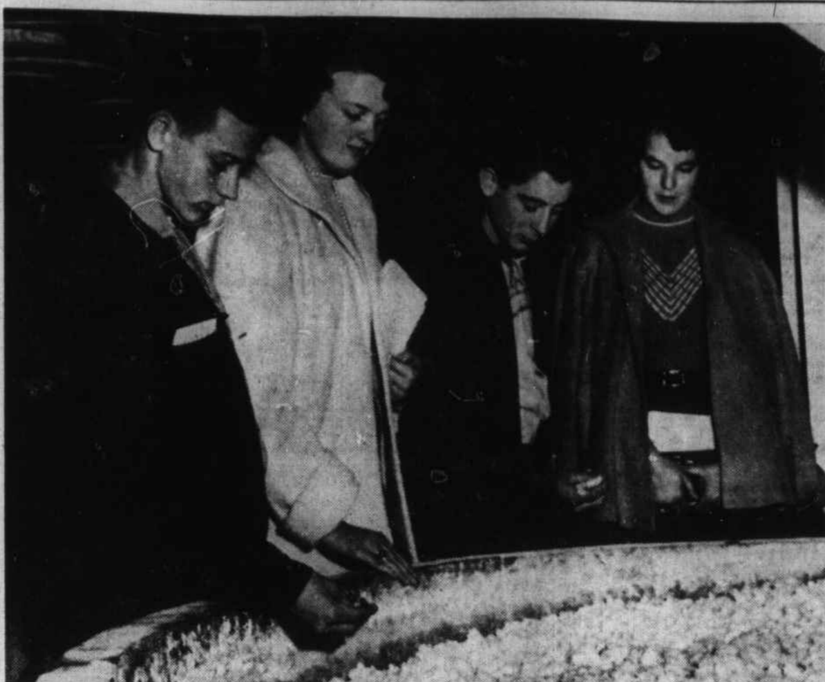
BETHEL SENIORS found this board mill pulp beater interesting as they toured the plant Wednesday about 64 strong. Left to right are Hoyt Norris, Bobbie Jean Blaylock, Gilbert Massie and Eva Nell Henson. (Photo by J. Deaton).
