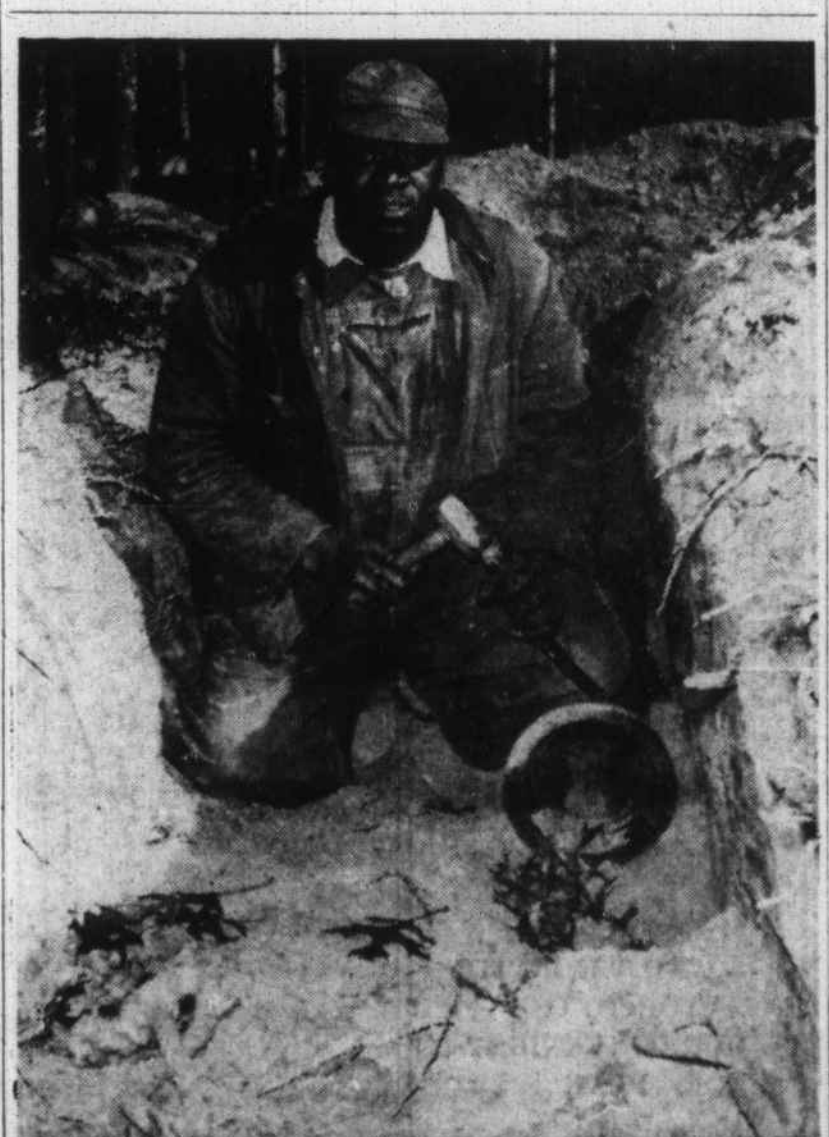
ED "EGG-EYE" ADAMS, observed his 30th year with the Waynesville Water Department Saturday. Here Ed is shown installing a 6-inch water main on the East Street extension line. (Mountaineer Photo.)
