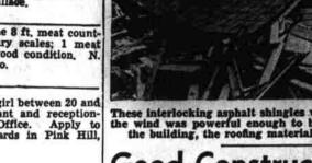
These interlocking asphalt shingles were properly applied. Although the wind was powerful enough to blow the complete roof deck off the building, the roofing material stayed in place undamaged. **Good Construction Defeats**
