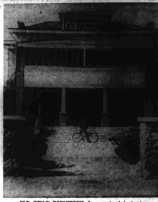
OLD GIRLS' DORMITORY—Is an outmoded structure in use since the Free Will Baptist Orphanage was established. Funds will be raised to replace the structure in the near future.
