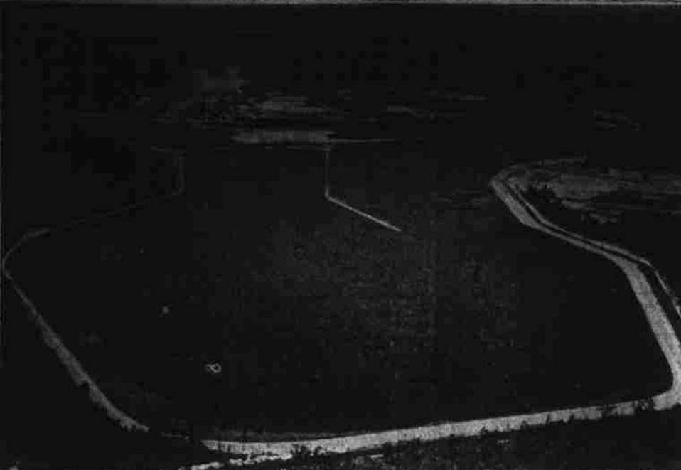
MAN-MADE LAKE COVERS 210 ACRES—This big lake near Lumberton has just been completed by Carolina Power & Light Company to cool water from its condensers before the water returns to Lumber River. It will protect sports fish from excessively warm water and will facilitate future expansion of the steam plant, engineers say. Senator Cutlar Moore of Lumberton sponsored a bill in the last legislature which made the big lake a waterfowl refuge.
