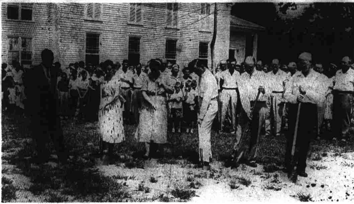
BREAKS GROUND FOR EDUCATION PLANT —With the pastor the Rev. U. A. McManus, Jr., extreme left in the foreground, and members of the congregation looking on, five members of the Bear Marsh Baptist church shovel dirt in breaking ground for the church's new education plant Sunday morning. Principals in the ground-breaking ceremony were, left to right: Mrs. Dorothy Nicholson, president of the Woman's Missionary Union; Mrs. Hazel Pipkin, training Union director; Elbert Davis, Sunday school superintendent; Leslie Southerland, finance secretary, and David Brock, chairman of the building committee.—Staff Photo by Vaden Brock.
