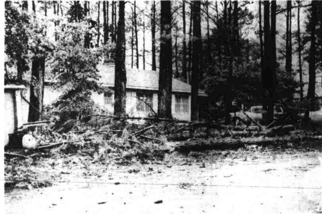
A view of the home of Mr. and Mrs. Philip Kretsch of Kenansville after a tornado wind passed through Kenansville on Wednesday morning.
