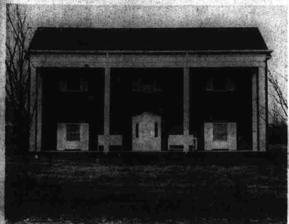
The Warsaw Masonic Lodge building No. 677 which was built during the year 1961. Open House will be held on Sunday, December 17 from Two O'clock until Five O'clock P. M. The
