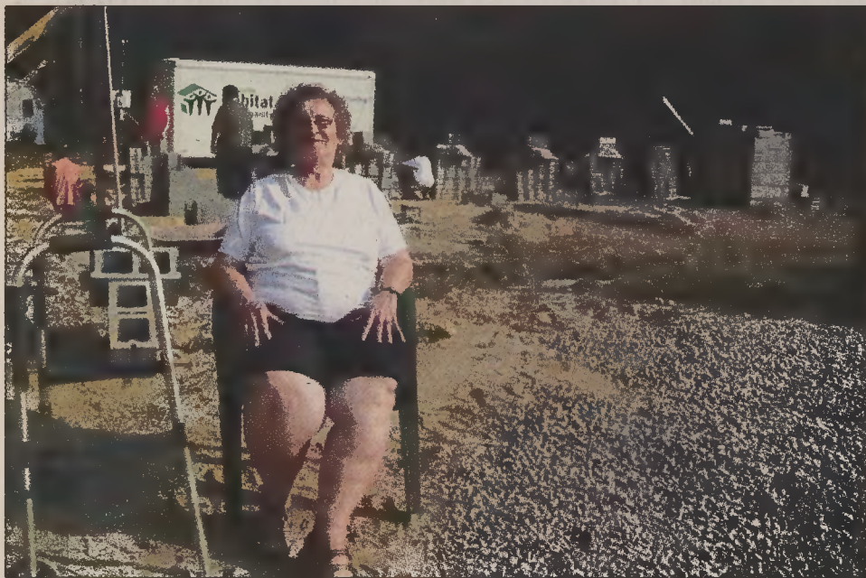
Virgil Morris sits on the lot where her home once stood as Habitat for Humanity volunteers work to build the foundation to her new house.
