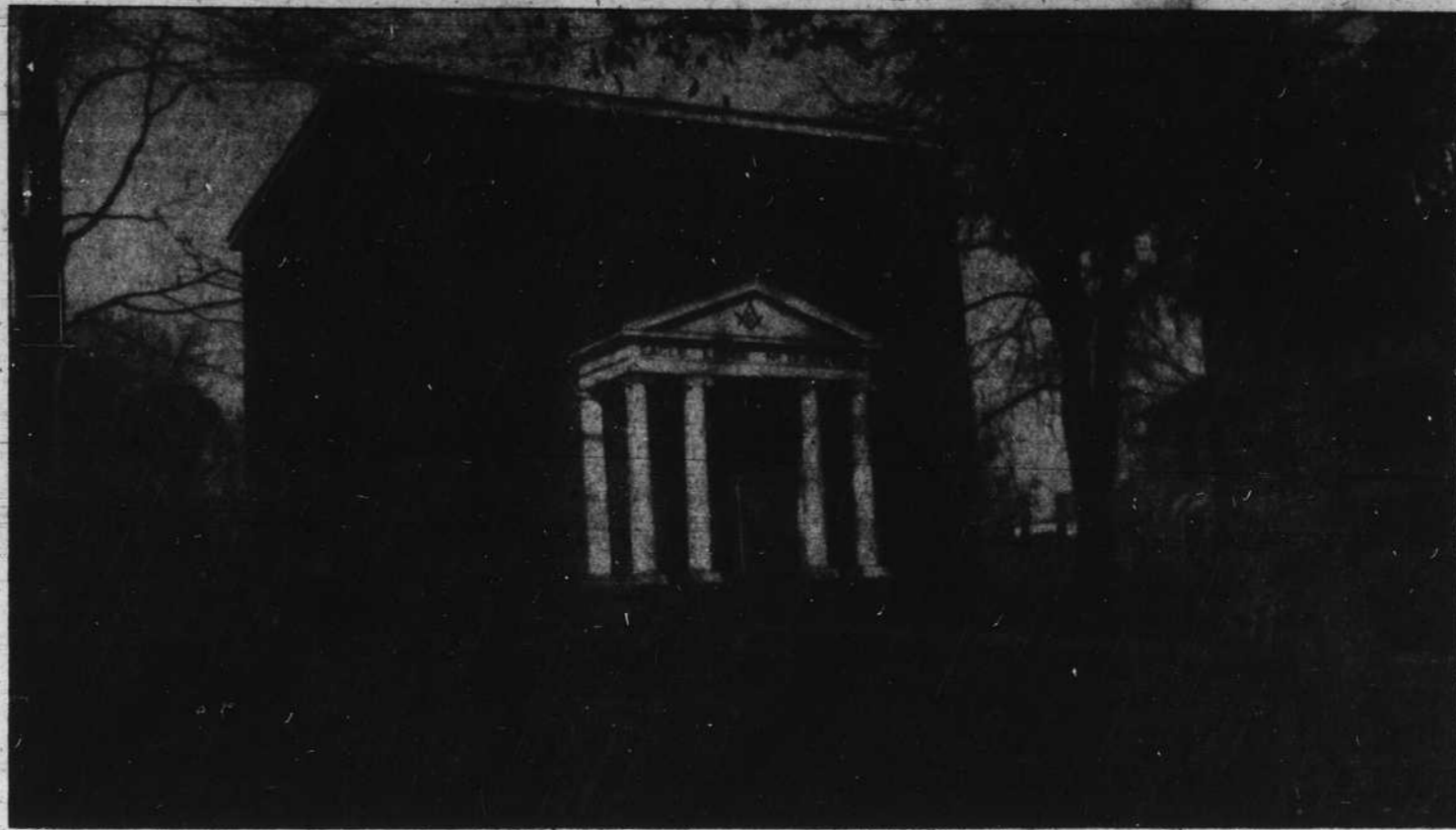
Eagle Lodge building at Hillsboro, that caught fire in the main room downstairs early last Tuesday morning. The blaze in the 122-year-old building was confined to the one room and was brought under control just before it burned into other parts of the structure. The building, constructed in 1823, suffered an estimated loss of about $2,000.
